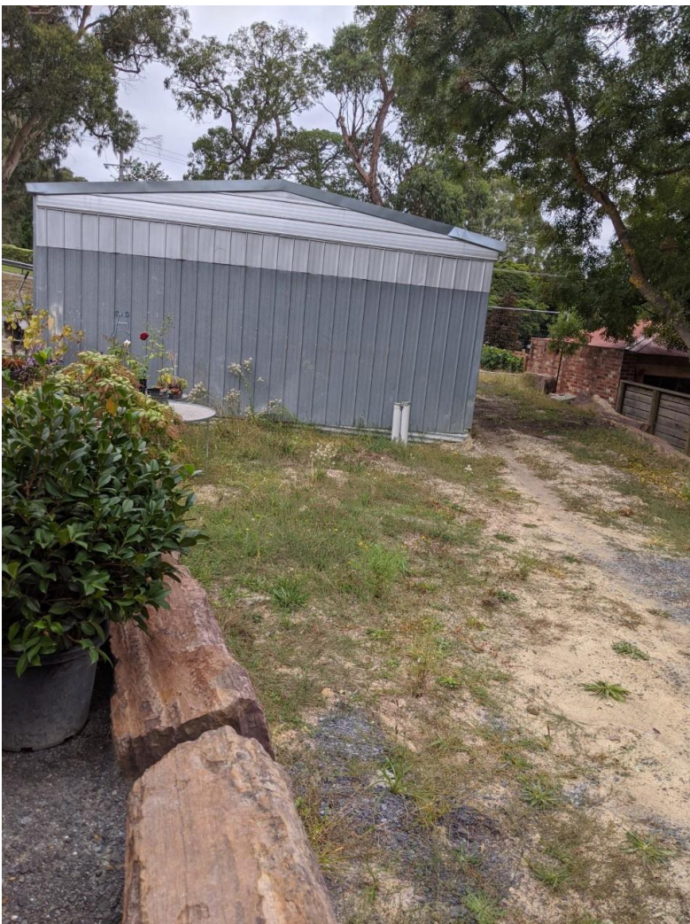
Figure 1. Rear of existing shed (Tapir, 2022)
